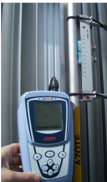
Measurement of nitrogen flow at pump outlet
